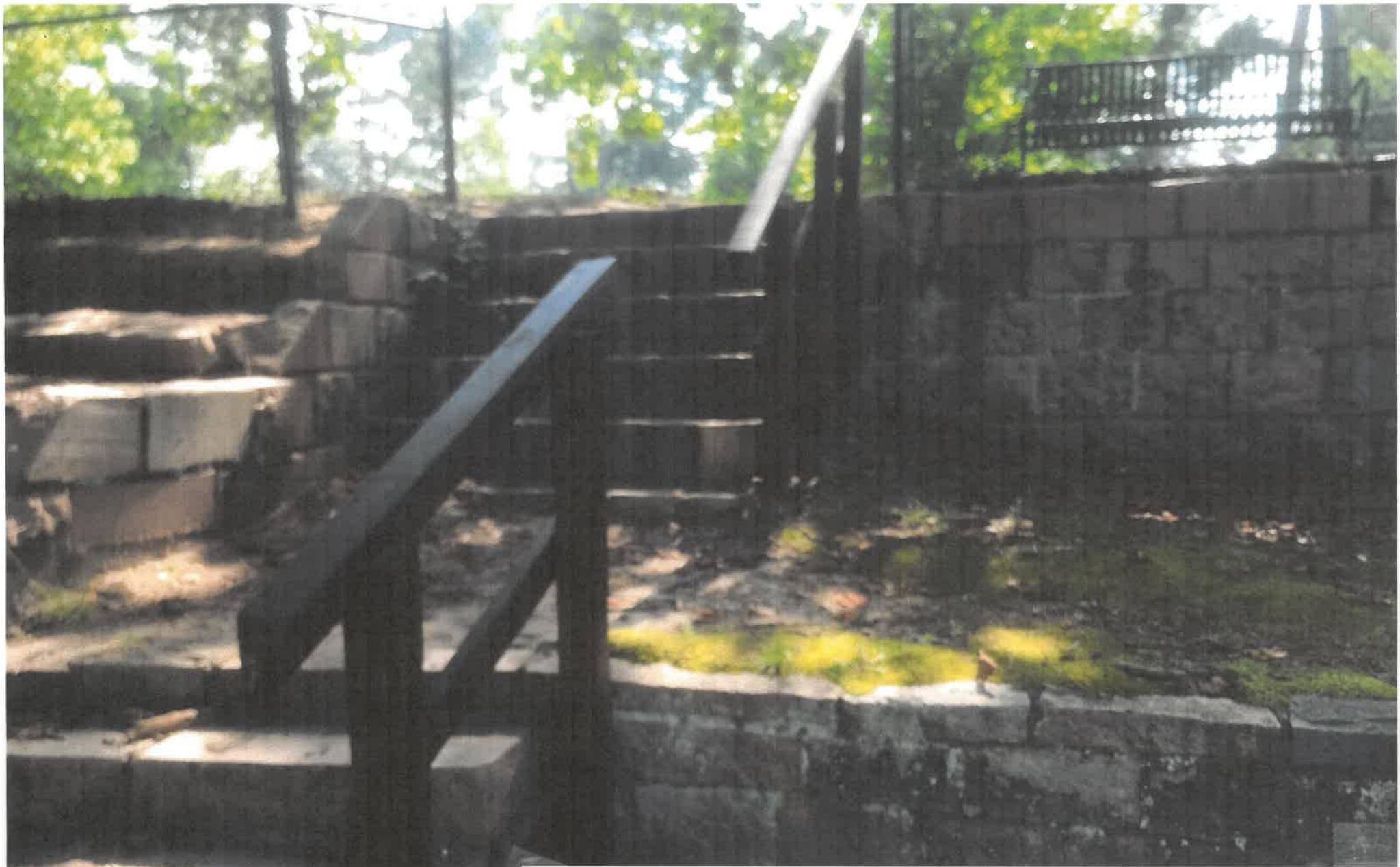
**Replace the wooden hand rails on both sides of steps with metal to match rails at shelter. The hand rails should connect with the fence at the higher elevation. Power wash steps and walls to the north.**
