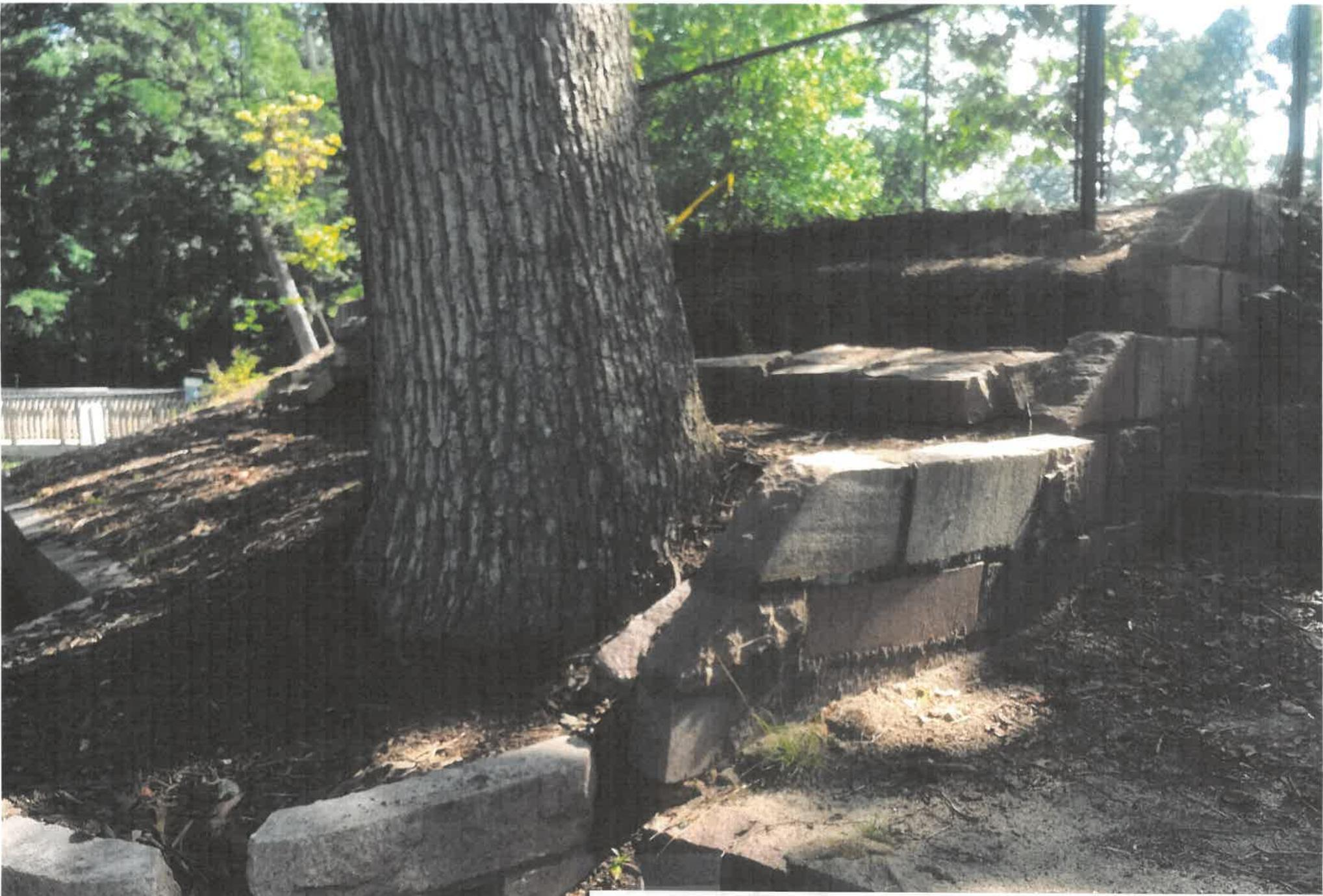
**Rework south side of steps before new hand railings are installed. Do not disturb roots of tree nor backfill at base of tree.**
